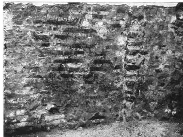
Fig. 149 — S. Lorenzo in Lucina. Right, core and internal brick face of original chancel wall. Left, secondary inner lining (Photo: Sansaini).
